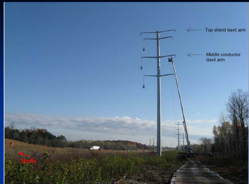
Figure 1 – Photograph of transmission pole 125 tested.
