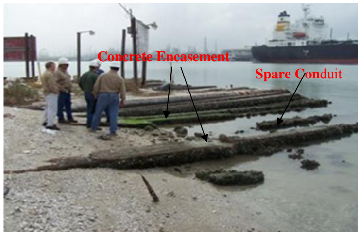
Figure 4: Locations of Encased Conduits
