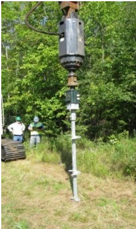
Figure 7. Three-Lead Helix.
