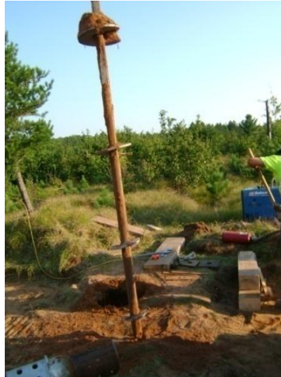
Figure 12. Four-helix Section.
