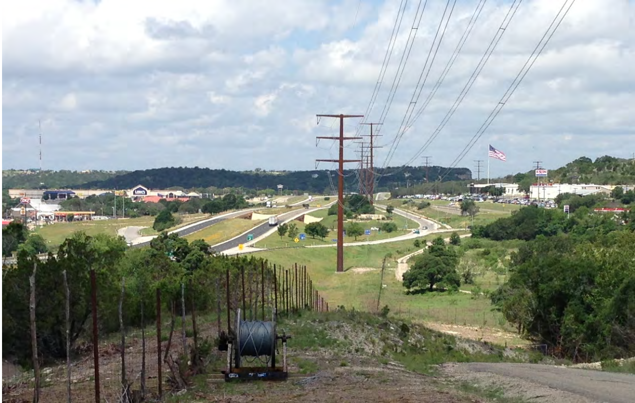
Figure 6: Big Hill to Kendall Transmission Line through Intersection, June 2013
